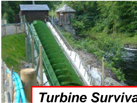
Archimedes Screw Turbines < 10 m head
