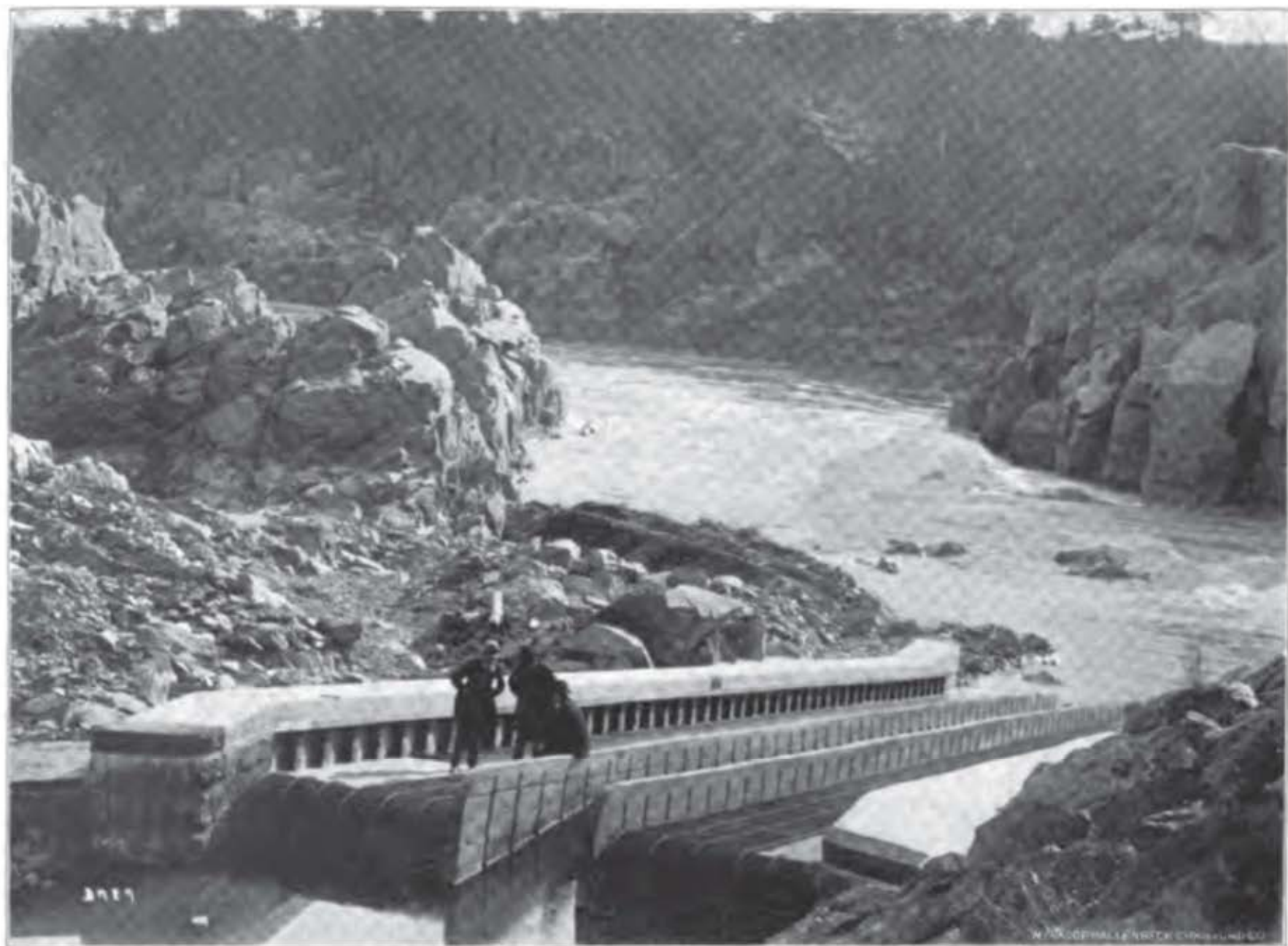
ORIGINAL McDONALD FISHWAY WITH WATER SHUT OFF, IN GREAT FALLS OF THE POTOMAC.
